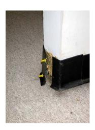
All construction work must be properly maintained, and sometimes individuals get creative in the techniques they use for this purpose. David Wyatt sent us this photo of a mechanical attachment that can be used in lieu of an adhesive for vinyl base. We suspect this photo was taken at an architect's office, based on the other photos that accompanied this one and the fact that a competent maintenance worker would never use push-pins. Duct tape or calk "yes," but never push-pins.
