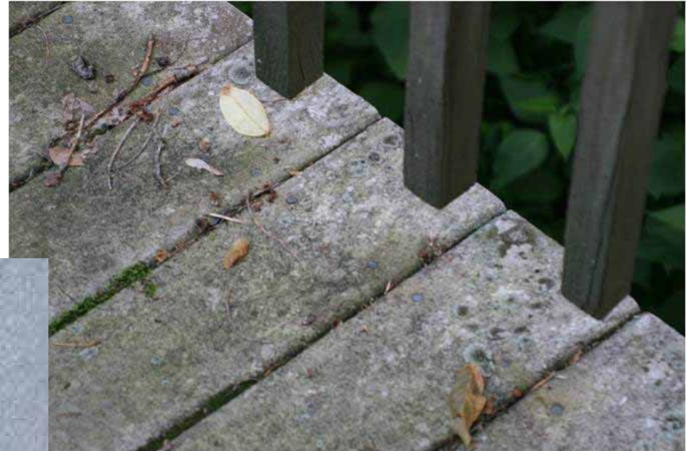
Mold on composite decking
