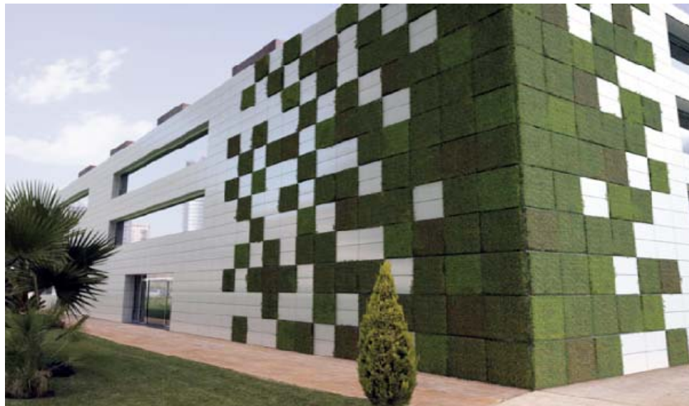
Vegetative panels inserted in a porcelain ventilated façade
