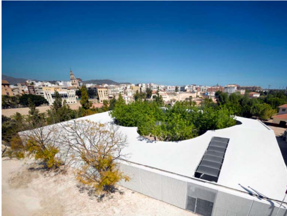
Elementary School - tile façade and roof, Gandia, Spain Photo credit: Paredes Pedrosa Arquitectos, www.paredespedrosa.com
