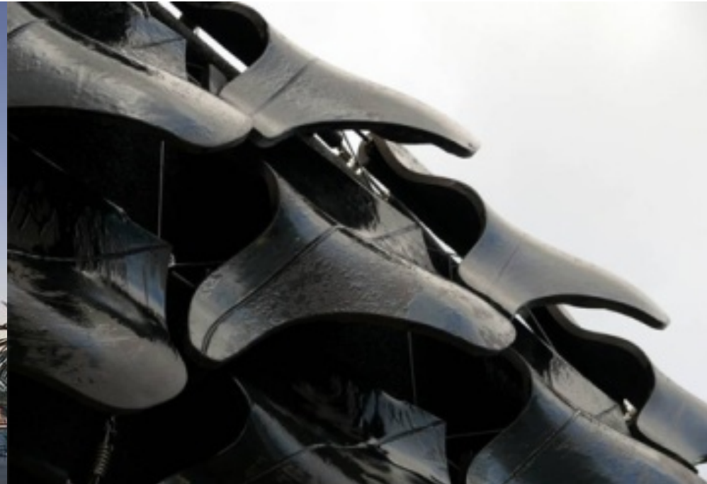
Villa Nurbs - façade Tile
