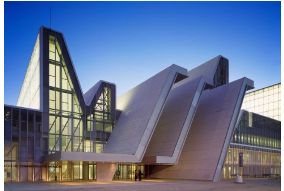
Congressional Palace - Tile and GFRC (glass fiber reinforced concrete) panel roof, 2008 Expo, Zaragoza, Spain
