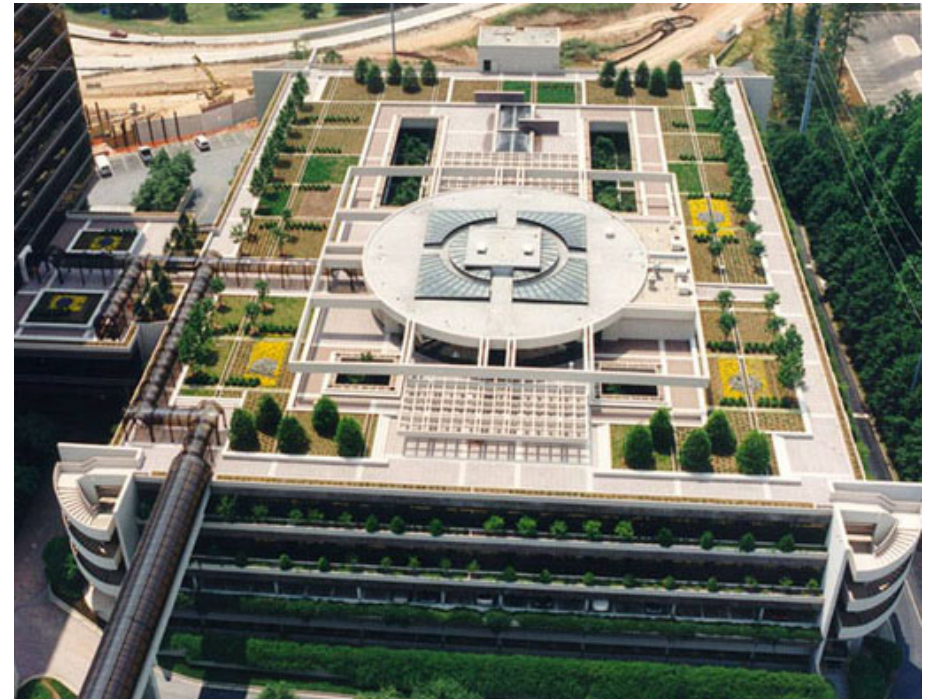
North Park 400 – Atlanta, GA Extensive and Intensive with Pavers
