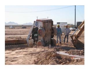
Foundation walls should always be properly backfilled and compacted. Otherwise, one might experience unexpected settlement. Experienced contractors always take care to ensure this work is performed in a workmanlike manner and always use the correct tools and equipment for this operation.
