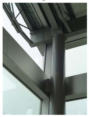
Here we see the architect that has chosen a very interesting glazing detail around a steel beam. Having carefully calculated the expansion and contraction characteristics of both the steel and the glass in accordance with normal temperature ranges, the architect has used his skill to design control joints to provide a design that celebrates the structure of the building. NOT!
