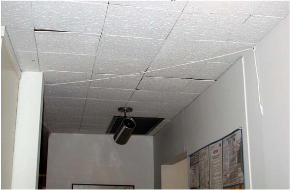
Here we see a typical installation of communication wiring prior to *MasterFormat* 2004. Now with the new Communications Division, this type of situation might be avoided with coordinated construction documents showing all work to be incorporated into the project.
