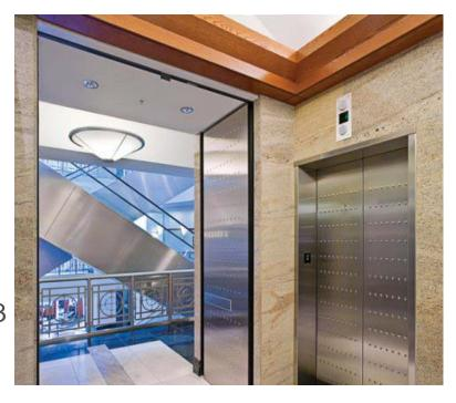
The elevator car door is fire rated but does not meet the Air Leakage rating and therefore does not meet UL 1784 requirements at this application.
