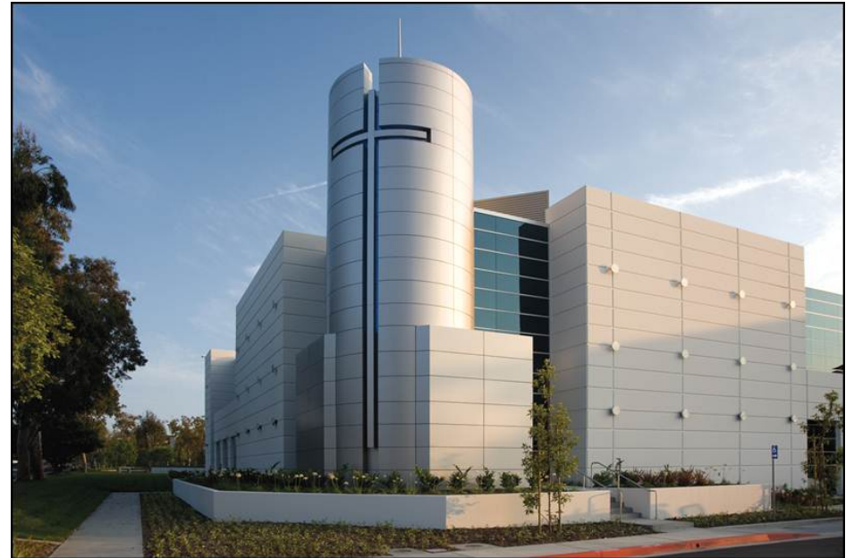
Bethel Korean Church, Irvine, CA Architect: Derevere & Associates Fabricator: Carvist
