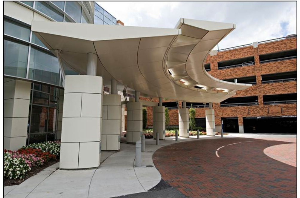
St. Mary's Medical Office Building, Richmond, VA Architect: Odell Associates Fabricator: W.H. Stovall
