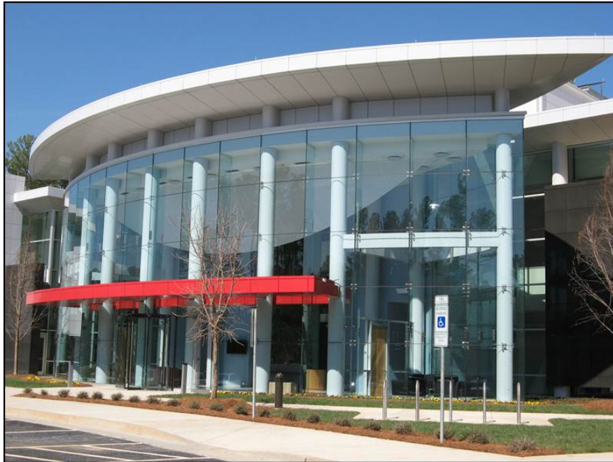
United Therapeutics, Durham, NC Architect: O'Neal Fabricator: Altech Panel Systems
