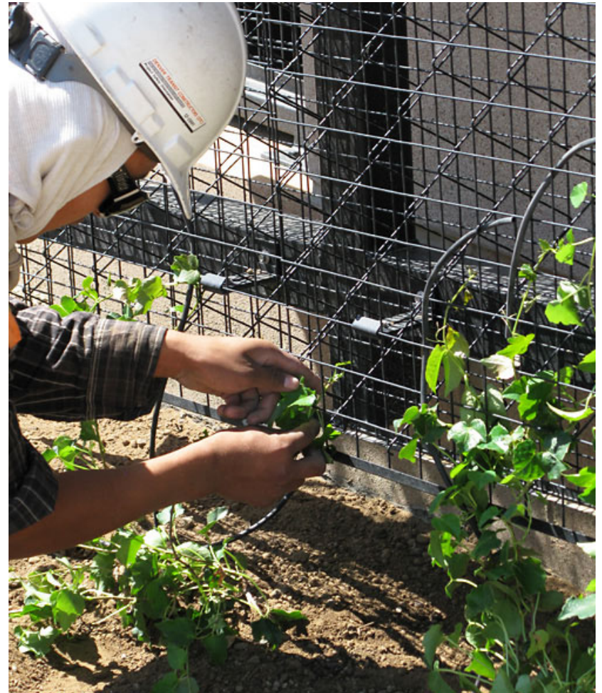
Proper plant installation and irrigation placement are critical to the success of green facade systems and should be inspected upon completion, Golden, CO.
