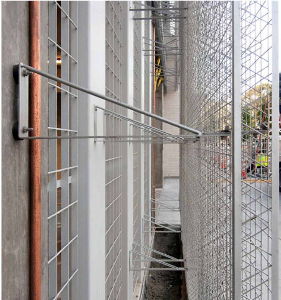
Wall-mounted, modular, three-dimensional panels with standoff brackets provide access to keep plants off the wall, Oakland, CA.
