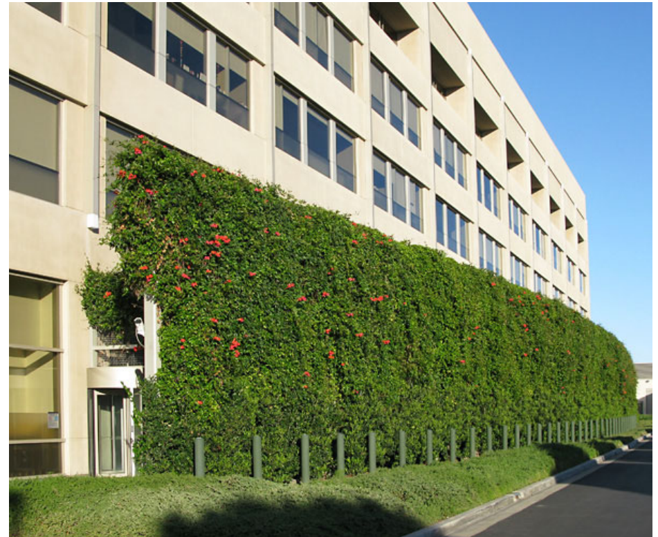
The first LEED® for New Construction completed building in California uses extensive green facades, Irvine, CA.
