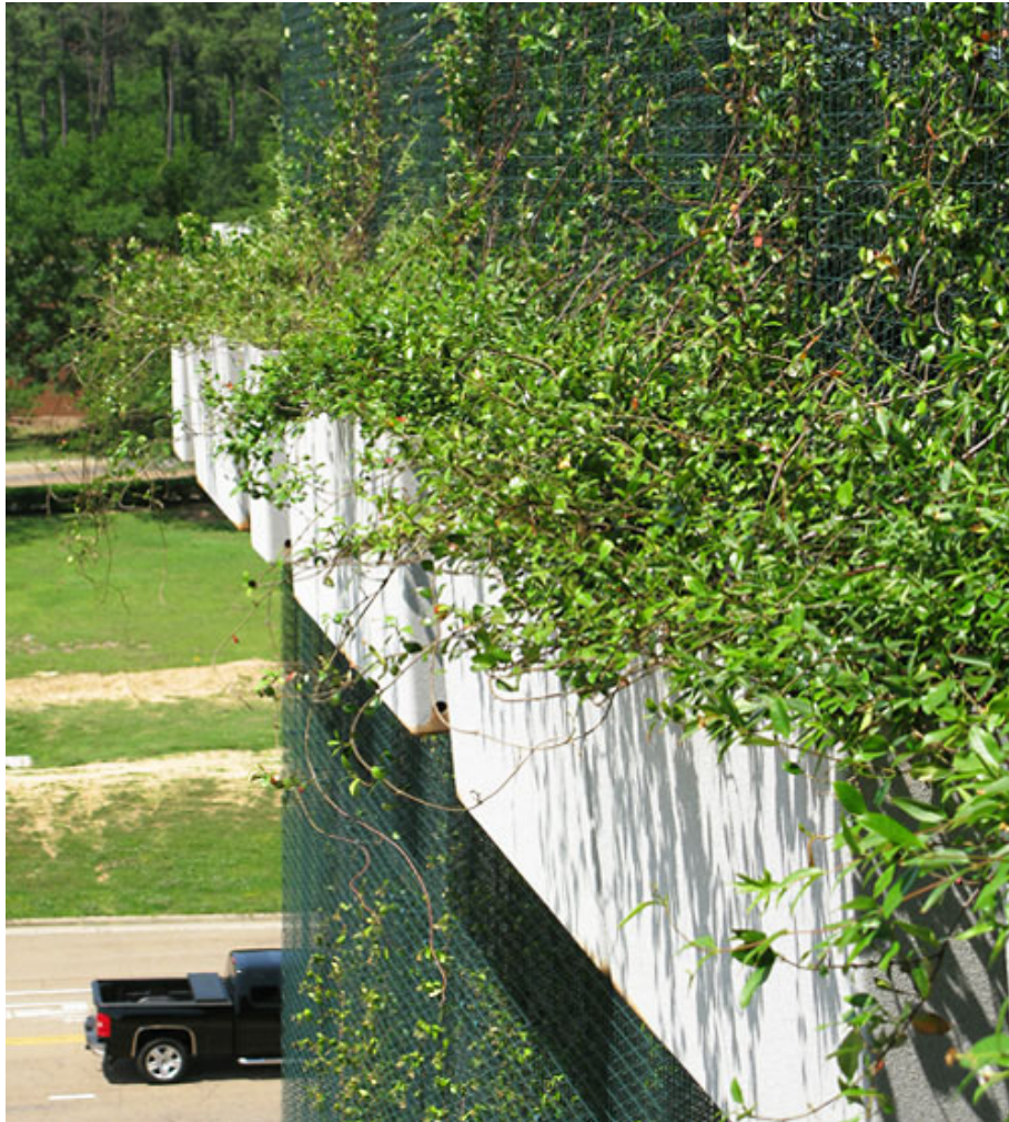
Planters with irrigation and drainage mounted to multi-level parking structure, Ridgeland, MS.
