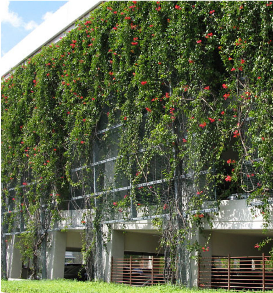
These vines planted directly into the ground have ample soil volume and correct spacing for full coverage to four stories, Fullerton, CA.
