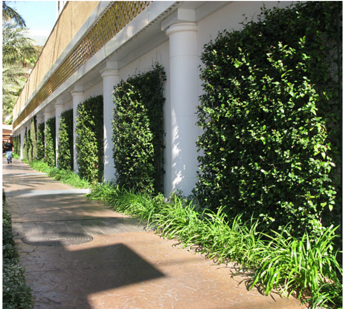
Multiple, three-dimensional panels with easy maintenance access help to reduce reflected light and heat gain in an arid environment, Las Vegas, NV.
