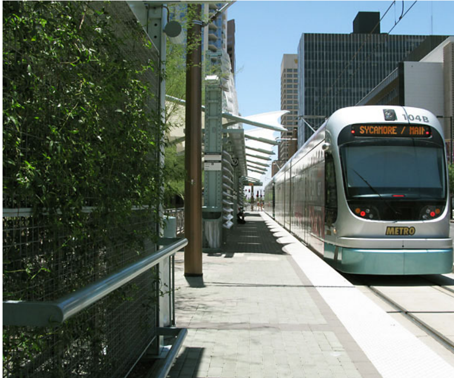
Green facades create shaded pedestrian areas and reduce UHI effects, Valley Metro Light Rail, Phoenix, AZ.
