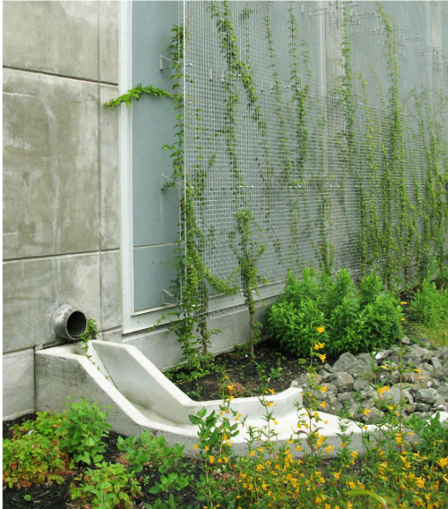
This rain garden with integrated green facade is a key component to the stormwater management strategy, Oakland, CA.
