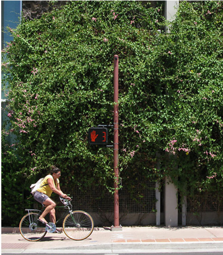
A green facade with climbing vines on a west-facing wall reduces the effects of an urban heat island on a sunny afternoon, Phoenix, AZ.
