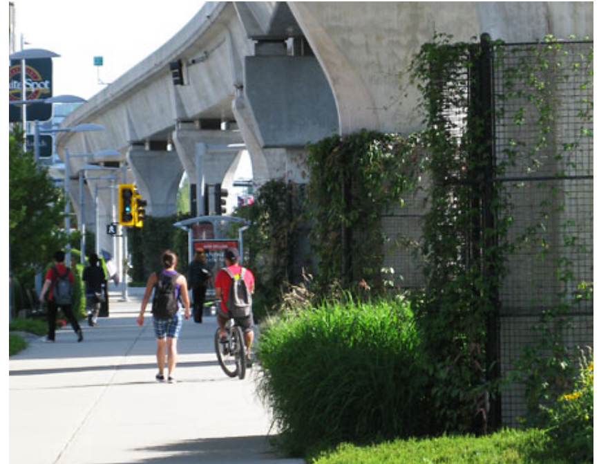
Green facade elements help with stormwater management and improve air quality, YVR Light Rail, Vancouver, B.C.
