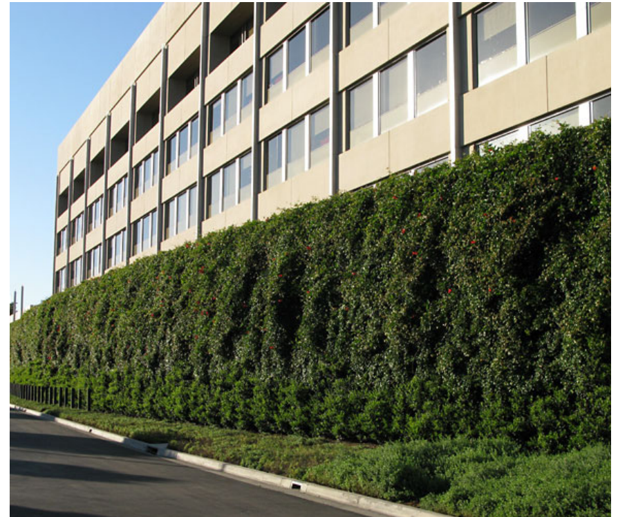
300 feet of freestanding green facade provides security, shade, and privacy screening, Irvine, CA.
