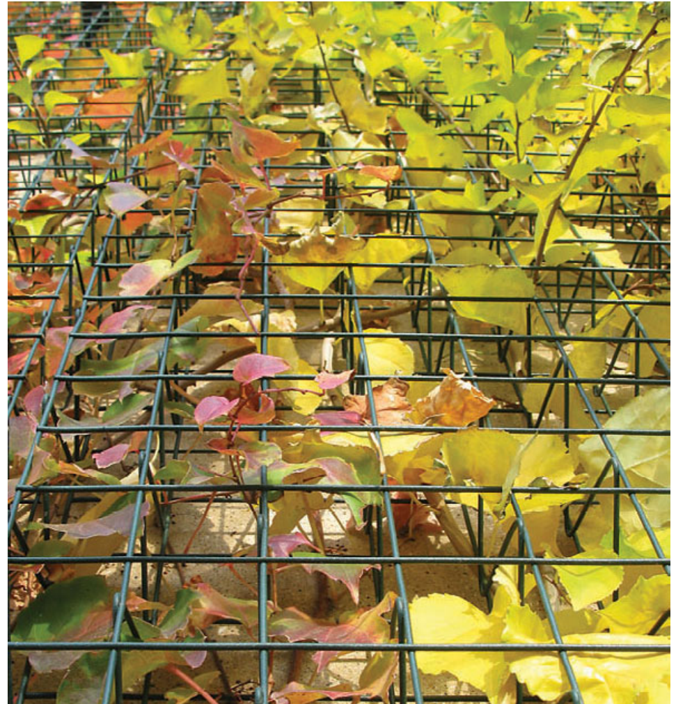
A wall-mounted, modular, three-dimensional, green facade system with plants showing seasonal interest, Chicago, IL.
