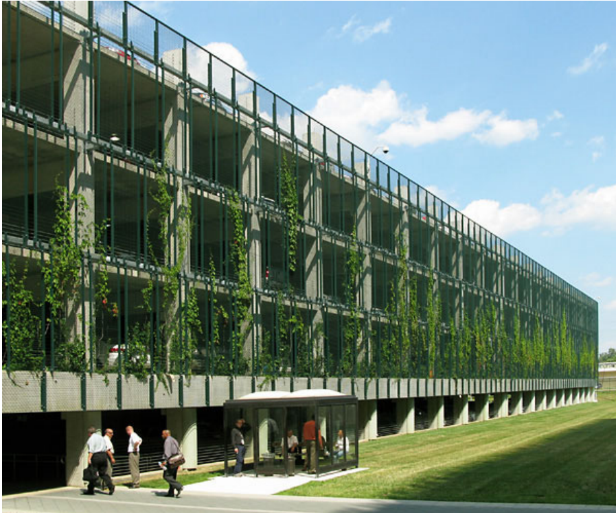
A parking structure with a green facade on all elevations utilizes elevated planters cast into the structure, Suitland, MD.
