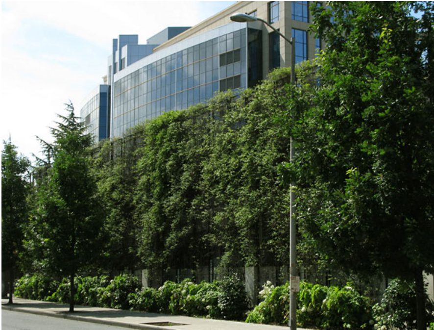
An east-facing, three-story, green facade attached to an urban parking structure, Seattle, WA.
