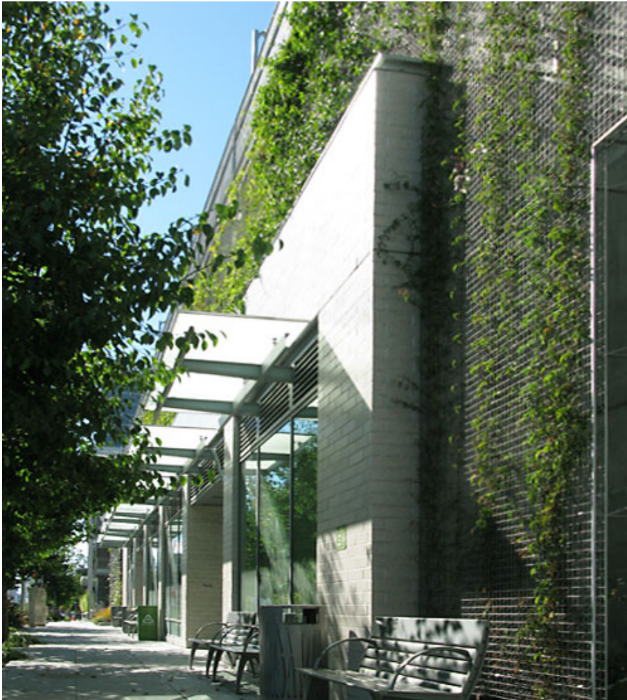
Matching attachment methods and fasteners to facade materials is critical for meeting exacting specifications, Oakland, CA.
