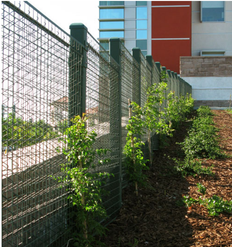
Green facade panels are incorporated into a freestanding fence for use as a wind break on this medical campus, San Mateo, CA.
