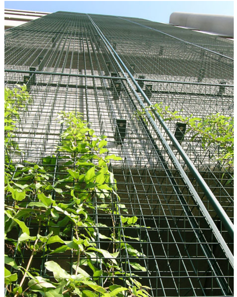
Six-story green facade with three-dimensional panels engineered for wind and snow loads, Rockville, MD.
