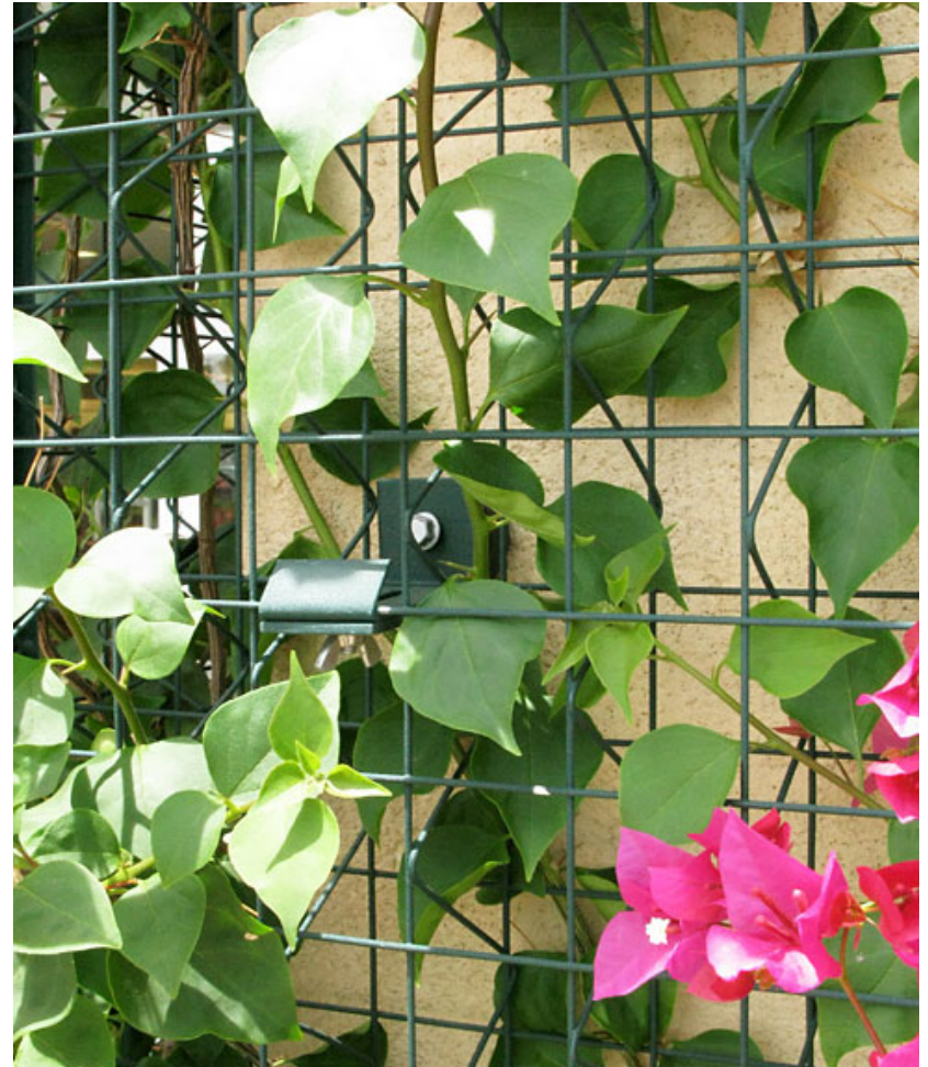
A panel mounting clip holds the facade panel off the building surface, and the depth of this three-dimensional panel system supports the climbing plant, AZ.
