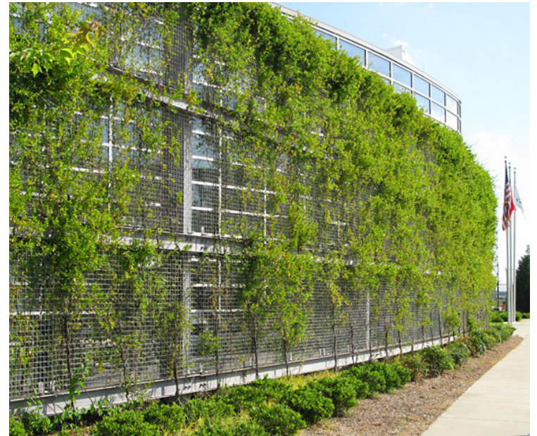
Regionally appropriate, native plant material installed with correct spacing begins to fill a freestanding green wall, Atlanta, GA.
