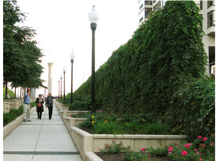
A freestanding green facade integrated into a green street demonstration project, Chicago, IL.
