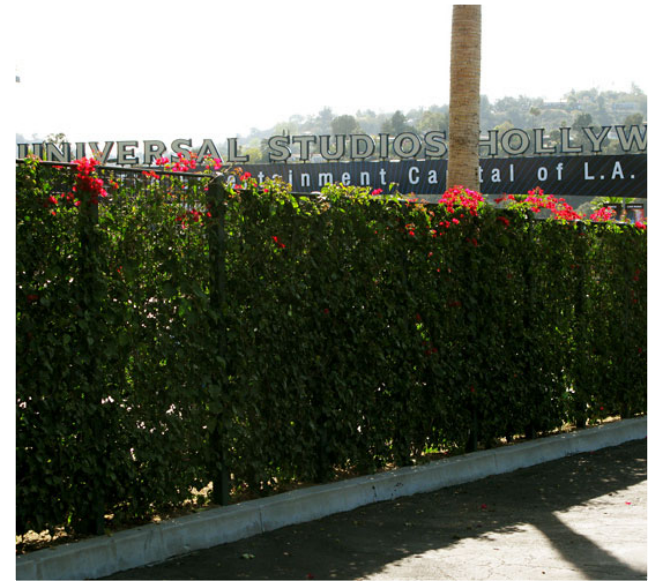
A well-maintained, freestanding application with a narrow planting area helps to screen views, define space and provide circulation control, Universal City, CA.
