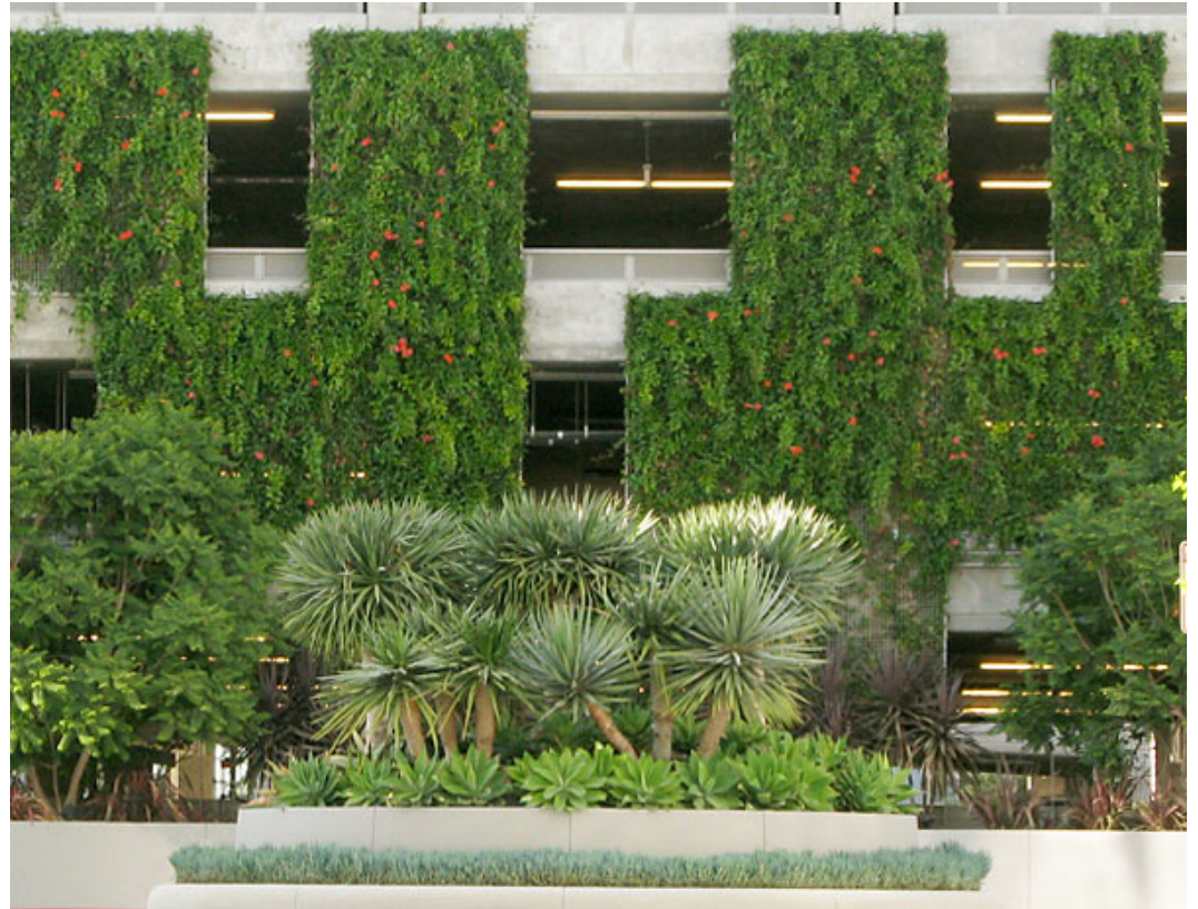
Surface-mounted green facade with plants trimmed to panel edges, Playa Vista, CA.
