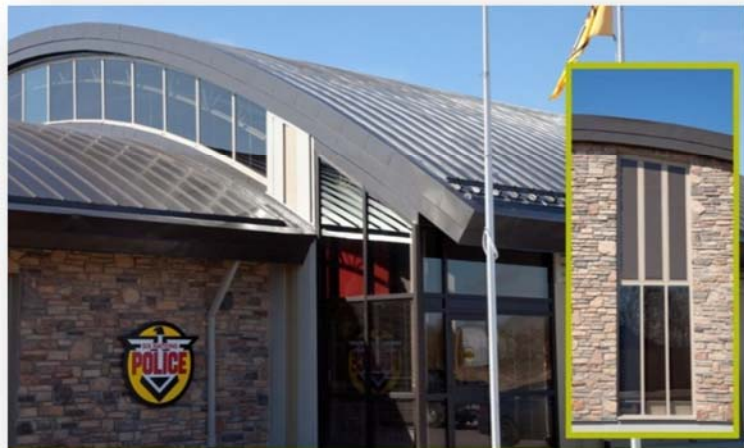
Six Nations Police Building, Ohsweken, ON
