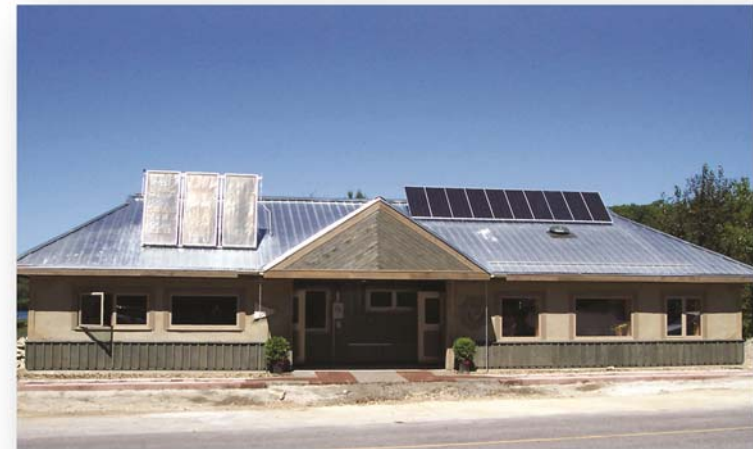
Sustainable Building by Fleming College, Haliburton, ON
