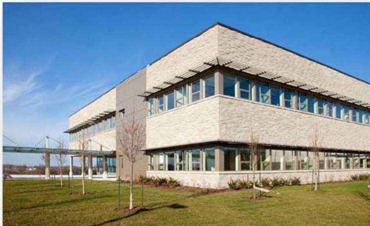
Waterloo North Hydro, Waterloo, ON
