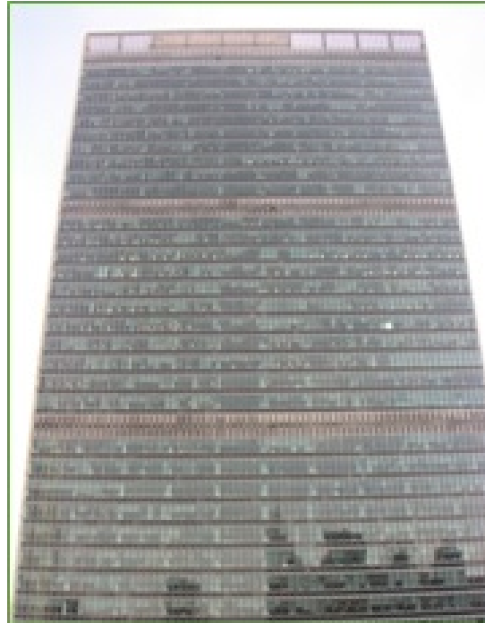
Checkerboard effect of blinds at various heights
