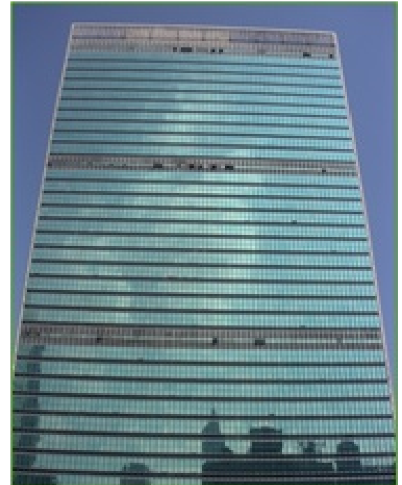
Window film providing a uniform look and reduced solar heat
