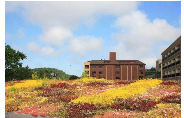
Hybrid Green Roof System: Grand Haven, Michigan, June 2008
