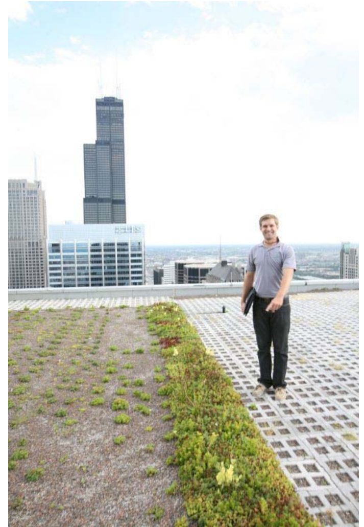
After a year of growing a plug-planted system (left) next to a pre-vegetated hybrid green roof system (right), the comparison demonstrated that wind scour is minimized and plant health is optimized by fully mature vegetation at the time of installation.
