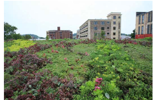
Hybrid Green Roof System: Grand Haven, Michigan, August 2007 (day of installation)
