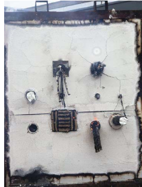
Exposed side of assembly frame. Note the cracks in the gypsum and the plastic that has melted away.
