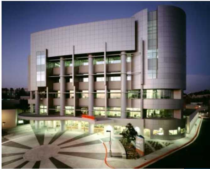
Sharp-Grossmont Hospital, La Mesa, California
