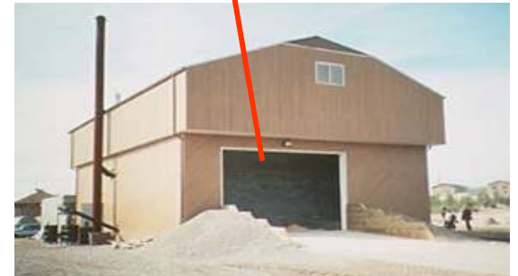
Ouje-Bougoumou, Quebec district system, burns waste woodchips from a local sawmill.
