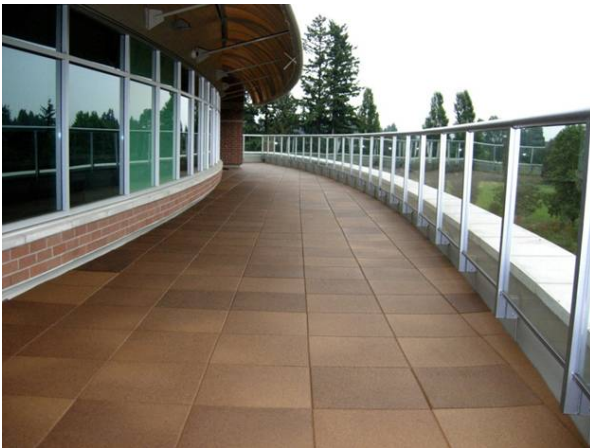
Elevated walkway with rubber tiles
