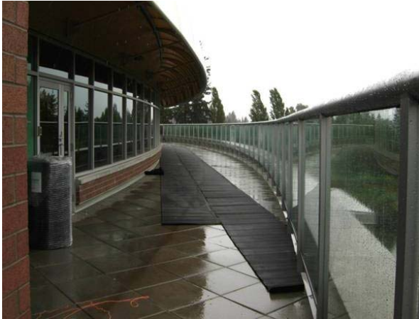
Elevated concrete walkway
