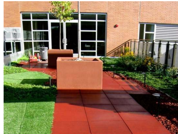
Rubber tiles used in green roof system
