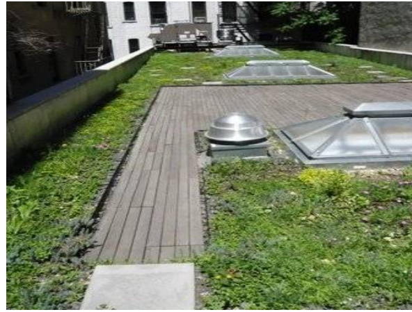
Wood decking used in green roof system
