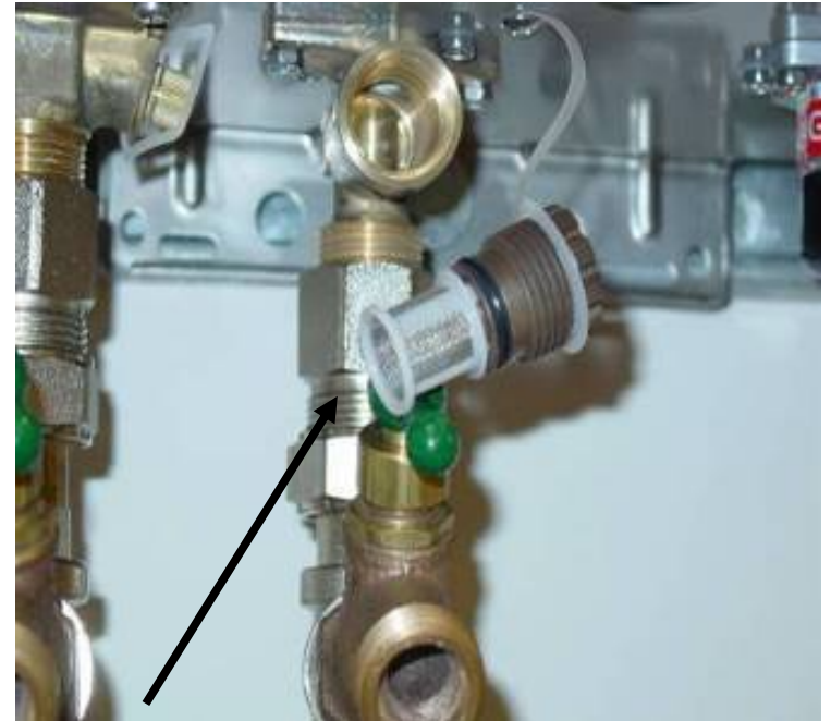
Water Filter - Before removing the filter for cleaning, ensure the water is turned off and the system has been drained by opening a hot water tap.
