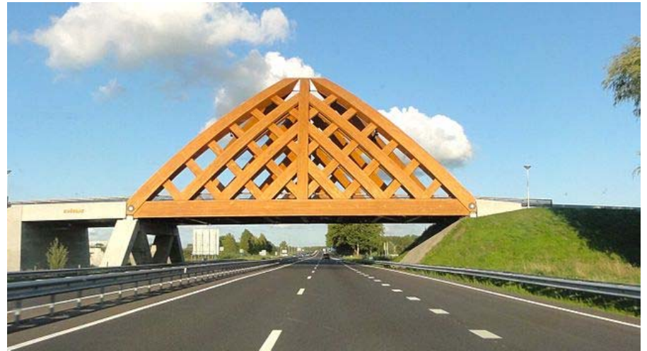
Acetylated wood bridge, Sneek, Netherlands
