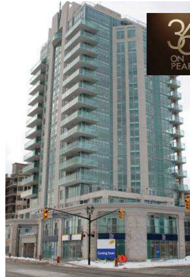
360 On Pearl 360 Pearl Street, Burlington, ON
