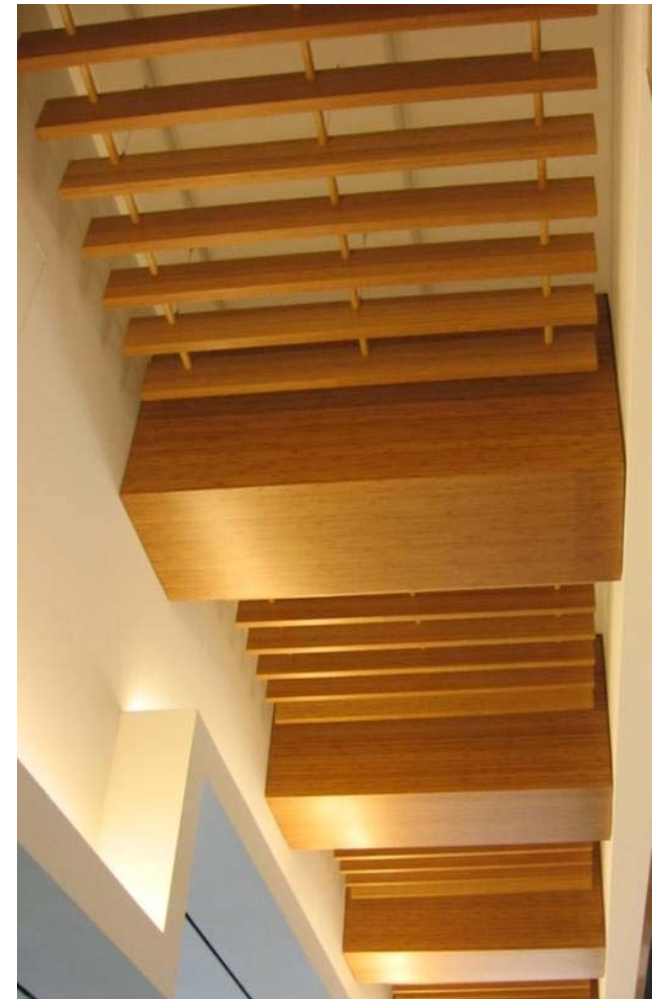
Custom Acoustic Ceiling Installation Using Traditional Bamboo Panels
