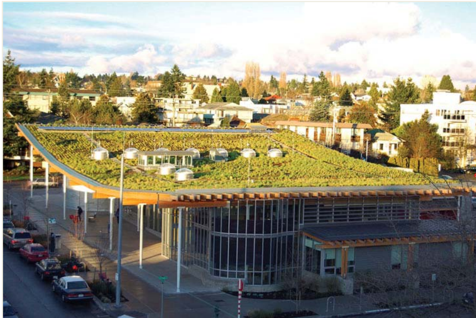
Ballard Library - Seattle, WA (sloped application)
