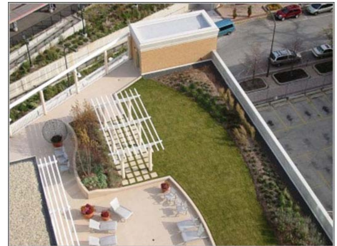
Church Street Station - Evanston, IL
