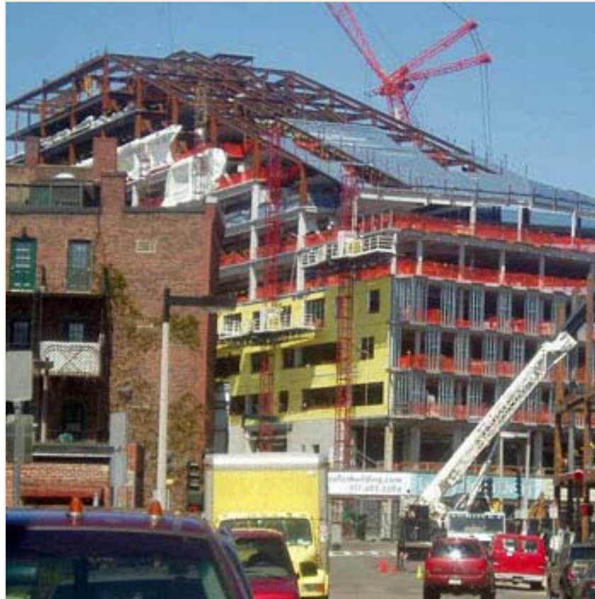
Macallen Building - Boston, MA
