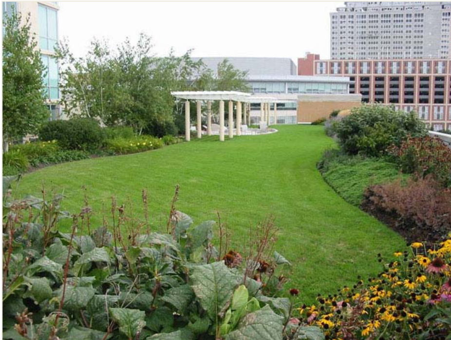
Church Street Station – Evanston, IL (over a 5 story parking structure adjacent to a condominium)
