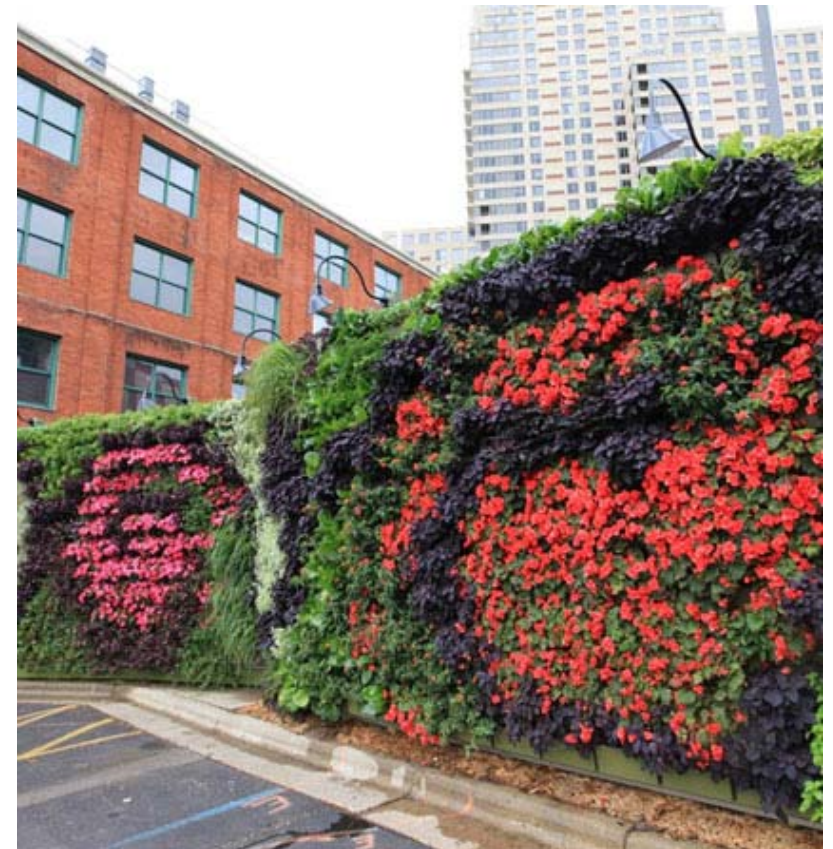
This living wall at the B.O.B. in Grand Rapids, MI buffers the noise and odors of the facility's necessary but unsightly dumpsters and HVAC units.
