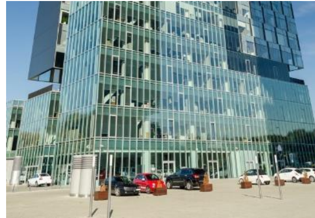
Getting to the building
